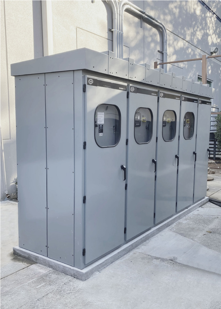
MCG Outdoor Paralleling Switchboard: installed onto concrete housekeeping pad
