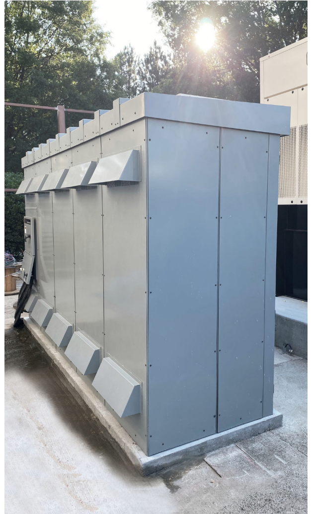
MCG Outdoor Paralleling Switchboard: installed onto concrete housekeeping pad
